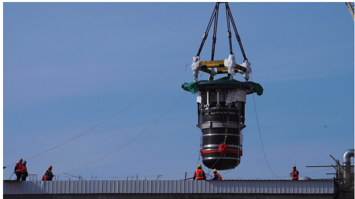
The reactor core being installed. (Photo: SIAP)
