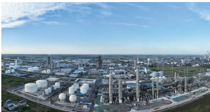
The world's largest 600,000 ton/year coal-based ethanol industrial unit.
