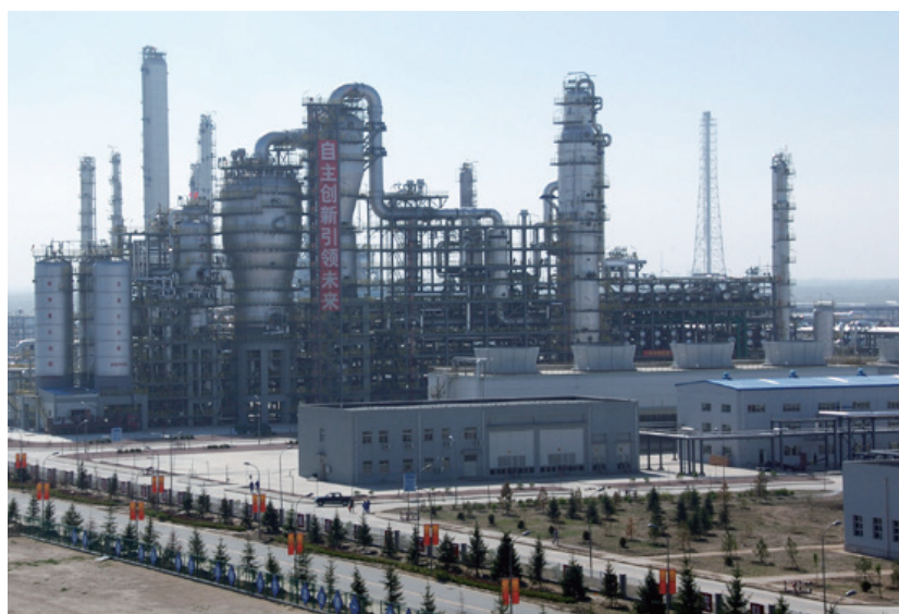
The world's first industrial methanol-to-olefins unit.
