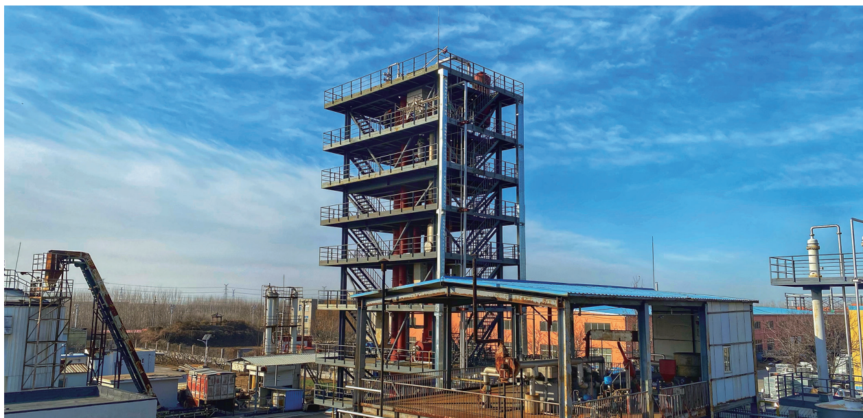
A 1,000-ton scale biomass chemical looping gasification pilot platform that produces green methanol.
