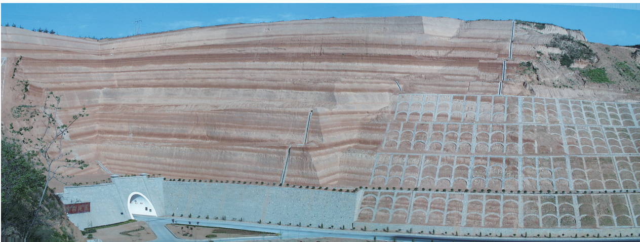
Fig. 2. The Outcrop of a well-known Chinese loess-paleosol sequence of the last 1.34 Ma with a thickness of ~85 m was exposed by Louzigou Tunnel highway construction in Tongchuan, a city near Xi'an, China. Brown-reddish and yellow-greyish layers in the photo show buried paleosols and eolian loess, respectively. The interbedded loess/paleosol layers indicate the alternating dominance of the East Asian winter and summer monsoons.
