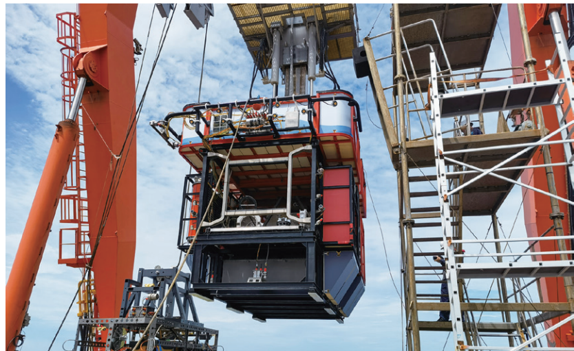
The first deep-sea energy storage system with megawatt-hour capacity are being employed for deep-sea operation.
