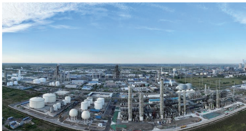
The world's largest 600,000 ton/year coal-based ethanol industrial unit.
